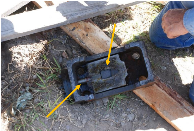
Box, wedge and adjustment nut and rod (yellow)
